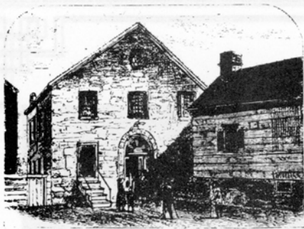
METHODIST CHURCH, JOHN STREET.
